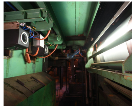
Figure 3 A SmartView system in operation on a pickling line
